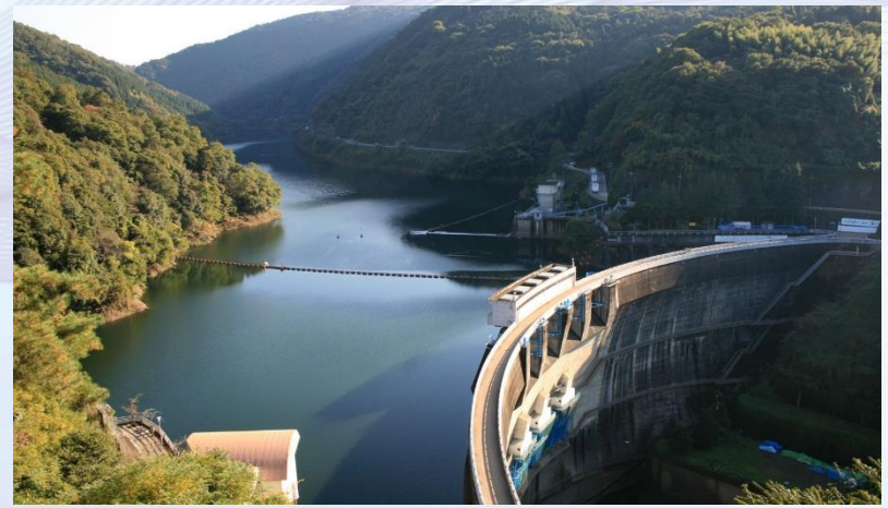
Suriname Afobaka Dam: 180MW
